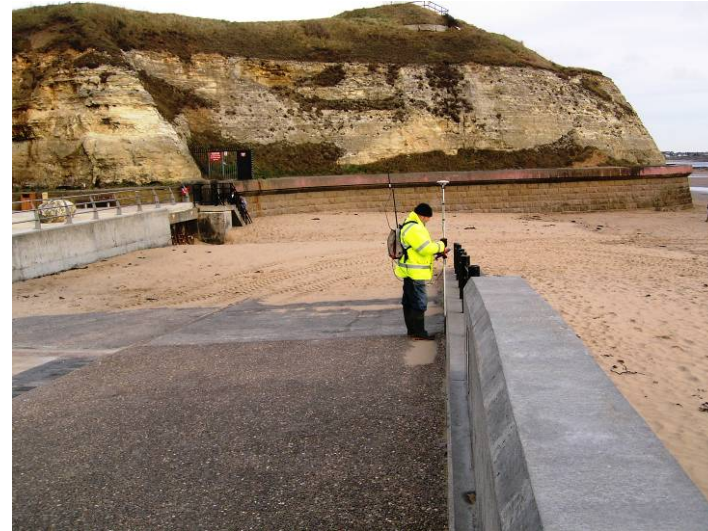
Plate 8 – Survey photograph 1bSNN10_20120320_N1.JPG (PM 2012)
