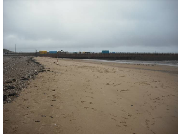
Plate 10 – Survey photograph 1bSNN12_20111013_N5.JPG (PM, 2011)
